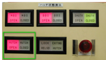
Hutch door is in opened condition
